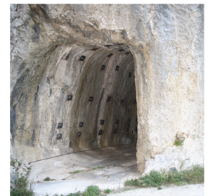
THE SMALL TUNNEL
